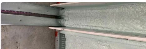
Z-bars with thermal breaks
