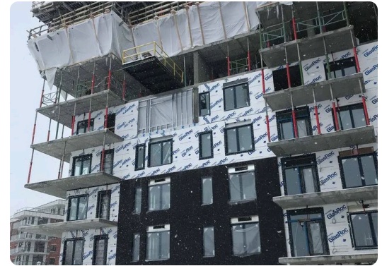
One building, three trades at once: cladding on floors 1–3, foam inside on 3–4, concrete on 6–7. Photo: Huntsman Building Solutions, D-Max Wall project.
