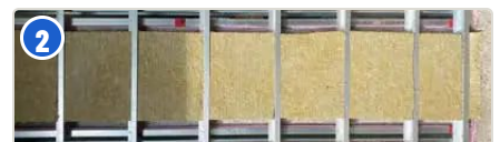
Sheathing On the Z-bars; mineral wool at slab edges
