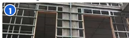
Studs and Z-bars On the outside face of the studs
